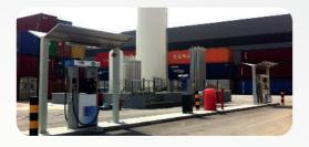
From the LNG, the installation allows the supply of both CNG and LNG.
